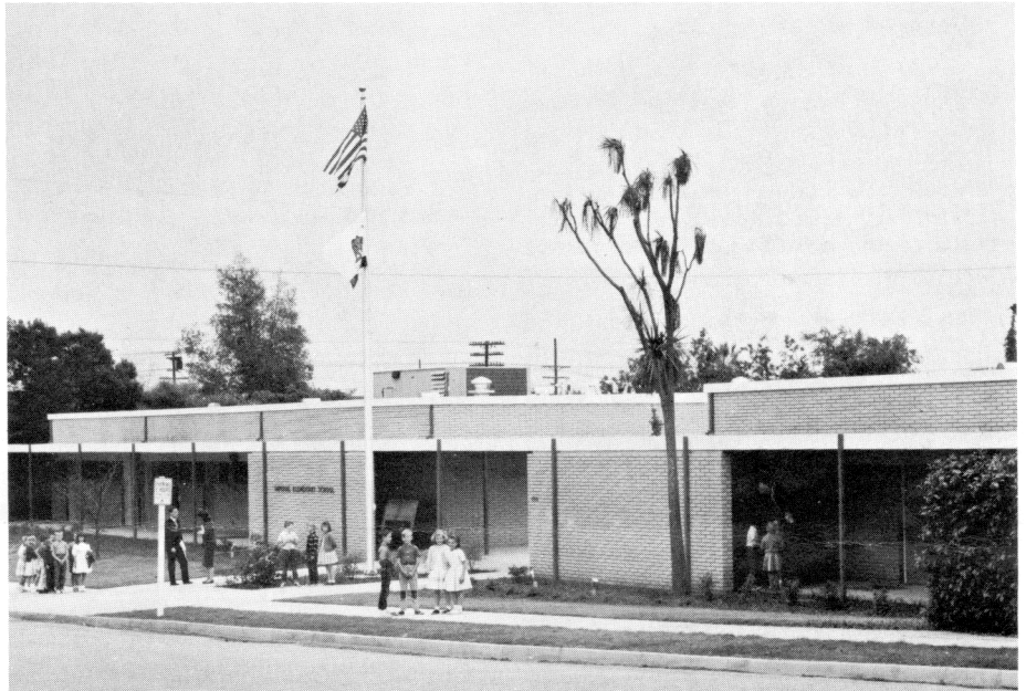
OUTSIDE—Attractive architecture and landscaping gives smiles to several students waiting in front of Imperial Elementary School.
